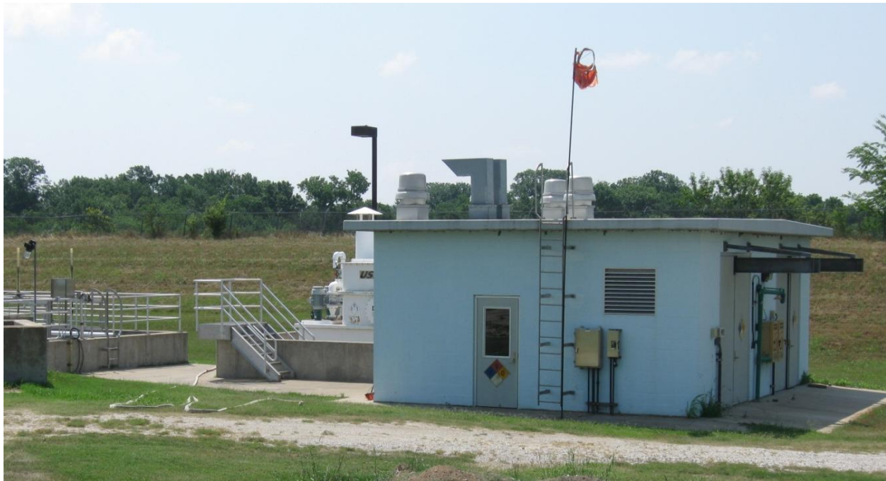
Figure 21: Chemical Storage Building and Scrubber Unit for Disinfection Process
