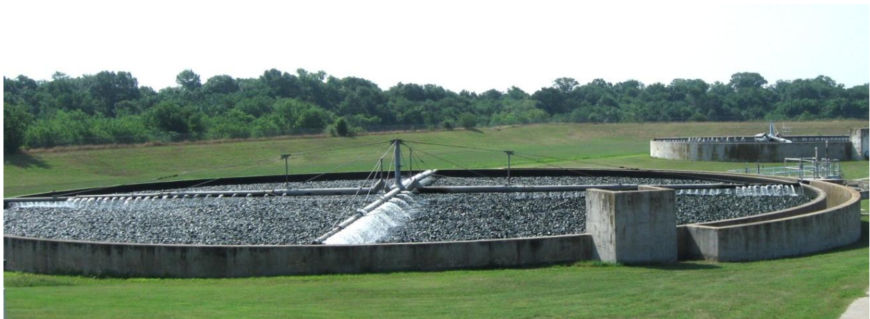
Figure 11: Stage 1 Trickling Filter
