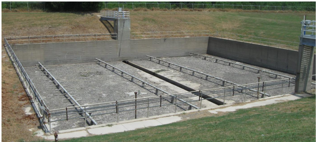
Figure 3: Equalization Basin at Front End of the Plant
