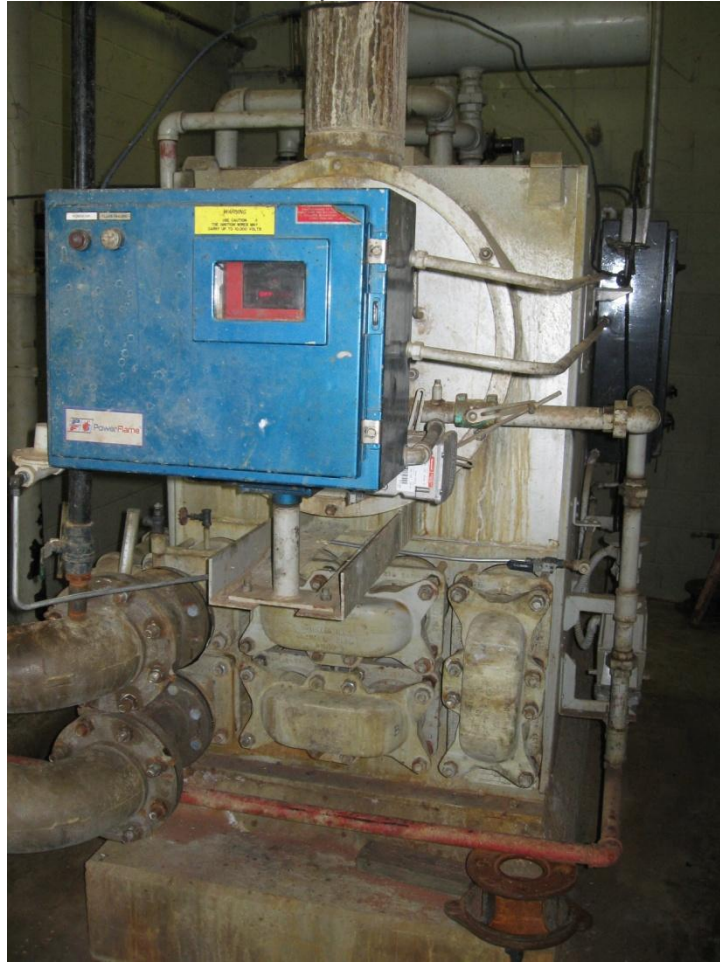
Figure 23: Heat Exchanger for Digesters Located in Solids Building
