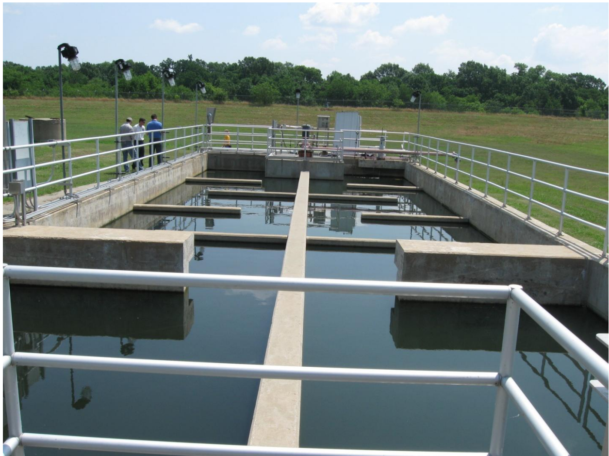
Figure 20: Chlorine Contact Basin
