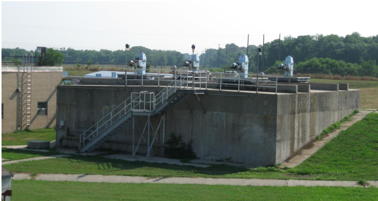
Figure 24: Anaerobic Digester with Mixers Mounted on Top Cover
