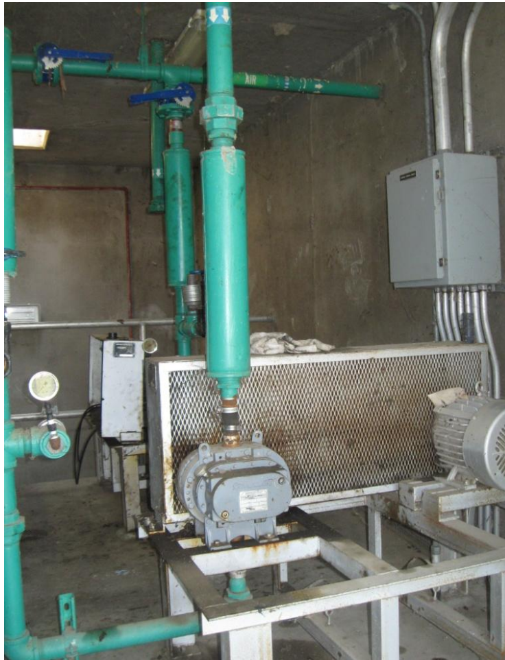
Figure 9: Blower Unit for Aeration of Grit Basins
