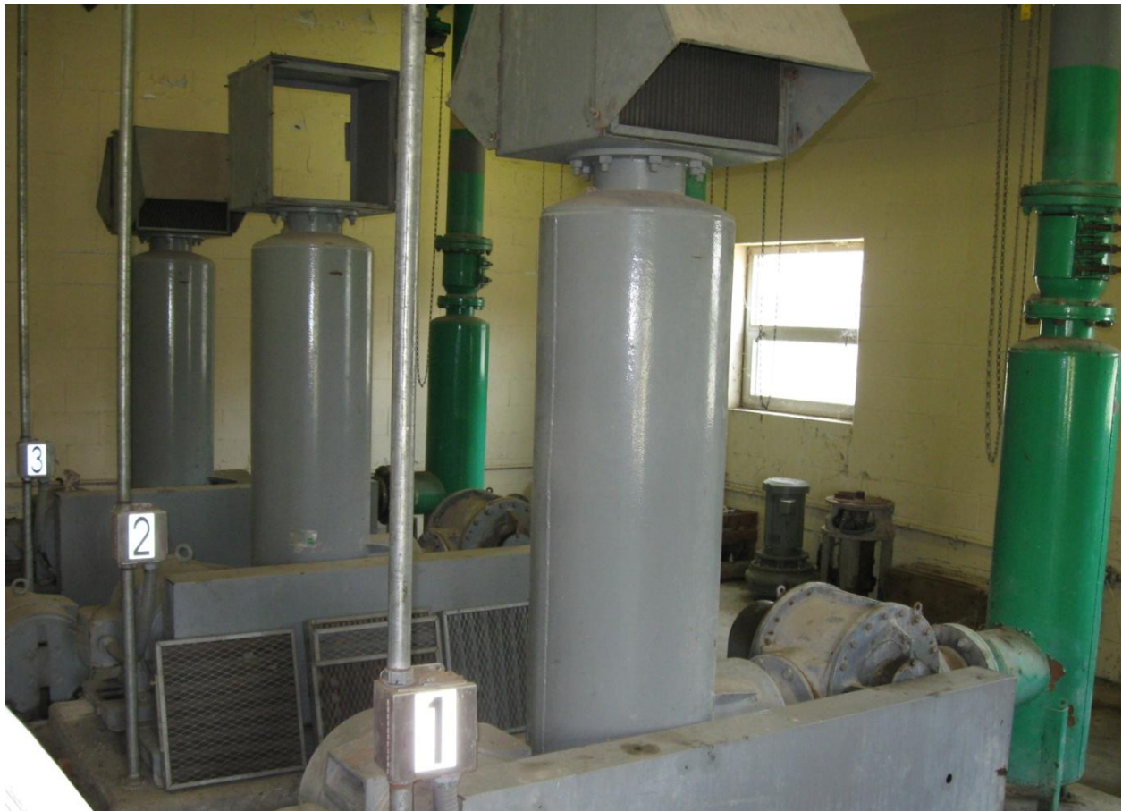
Figure 4: Blower Units for Equalization Basin
