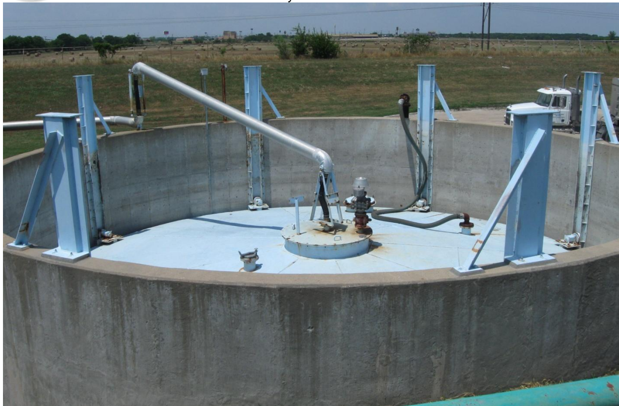
Figure 25: Sludge Holding Tank
