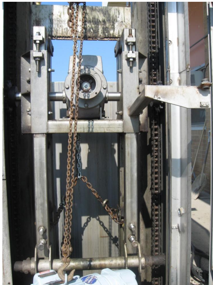
Figure 5: Motor and Lift Mechanism for Bar Screen Unit
