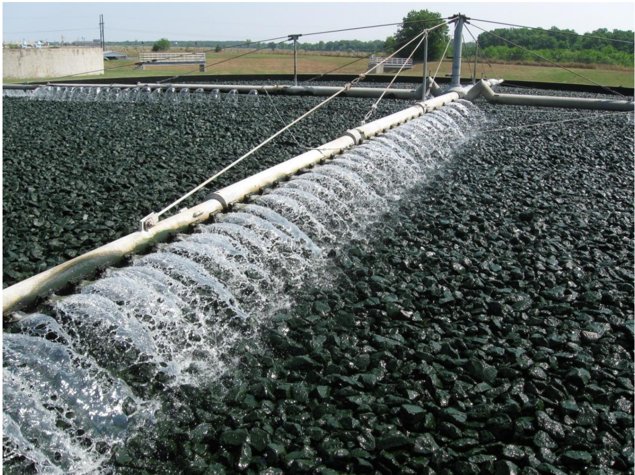
Figure 12: Distribution Arm and Rock Media of the Stage 1 Trickling Filter
