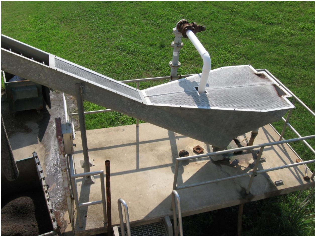
Figure 7: Grit Classifier and Washer Unit
