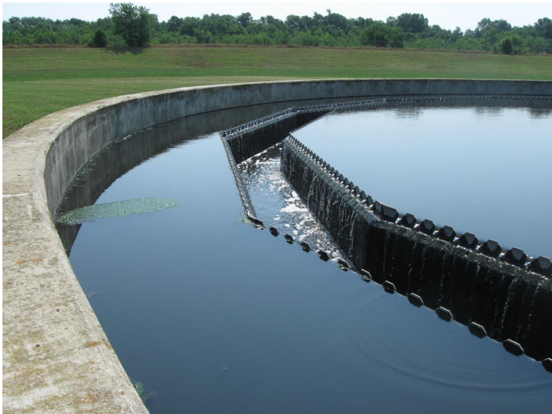
Figure 13: Intermediate Clarifier
