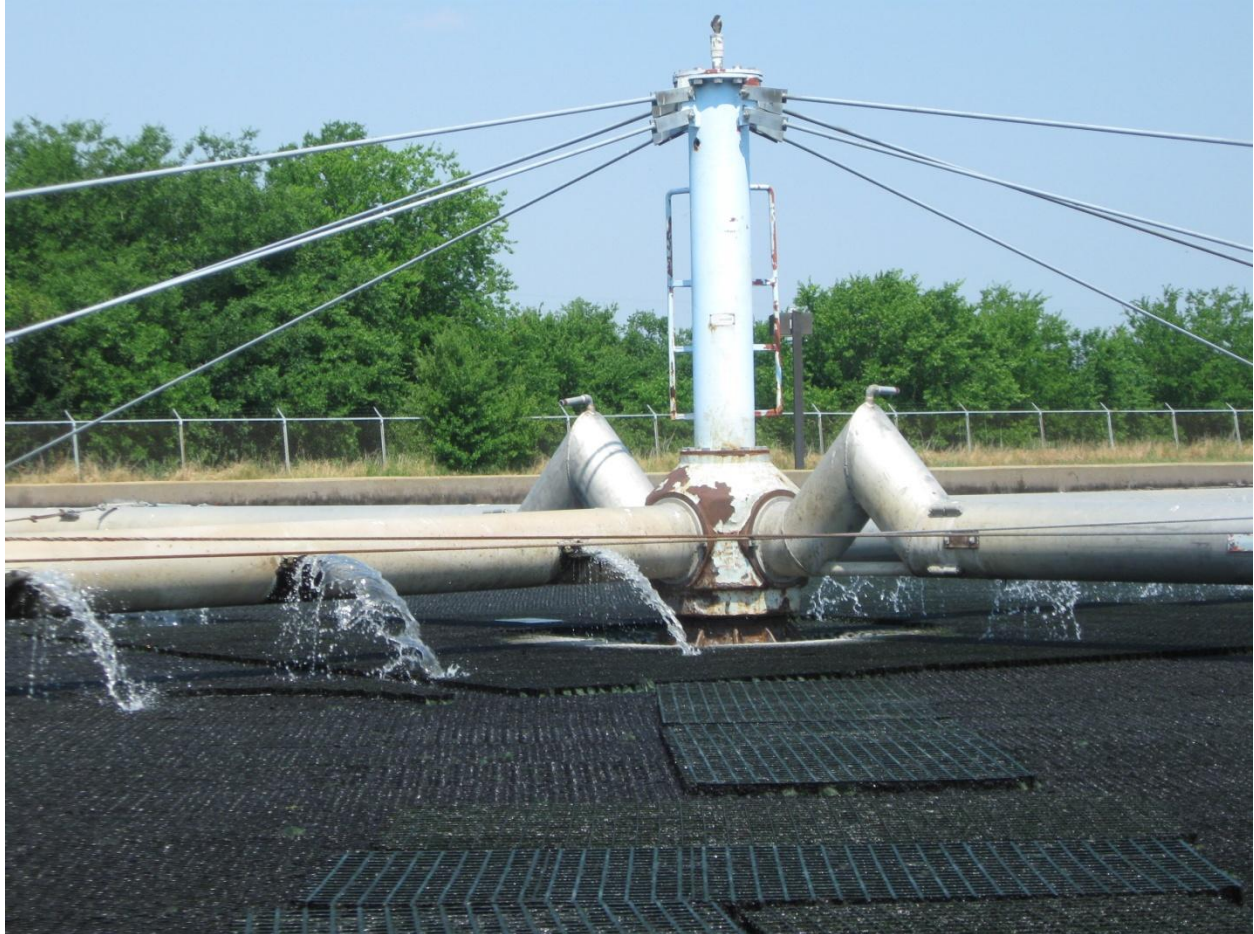
Figure 17: Distribution Arms and Brentwood Media of 2nd Stage Trickling Filter #2
