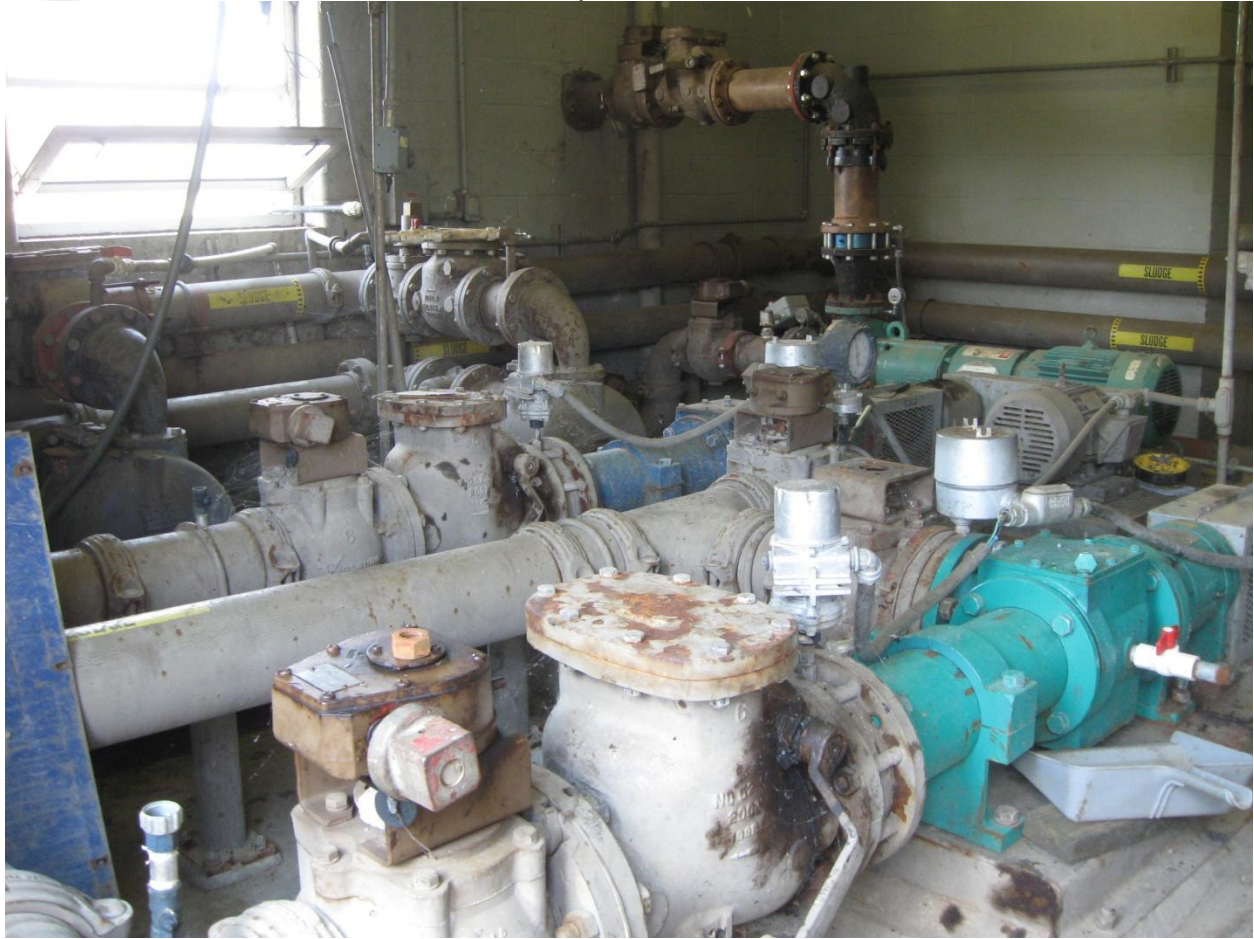
Figure 22: Sludge Pumps Located in the Solids Building
