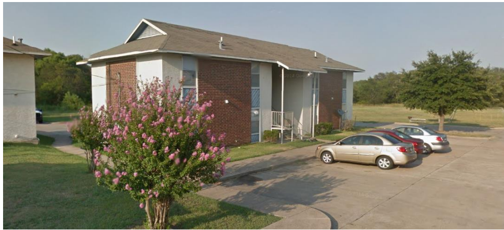
Undesirable - Inadequate Front Facade and Roof Articulation
