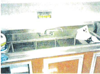
Three-compartment sink
